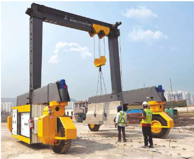
Handling of precast segments at a casting yard
